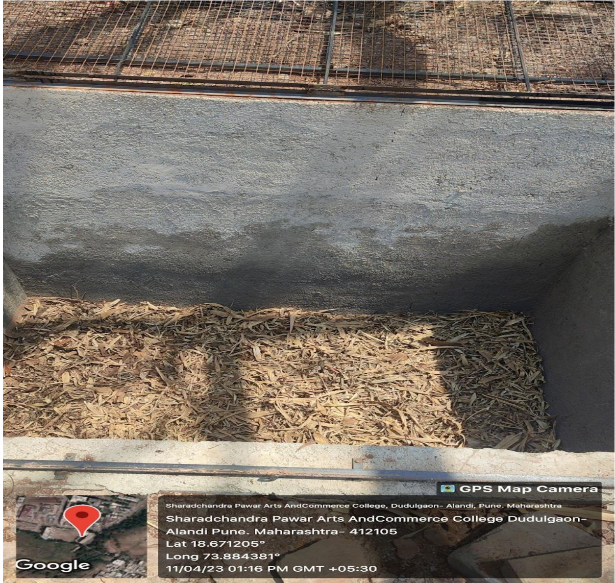
Solid Waste Disposal by Compost pit
